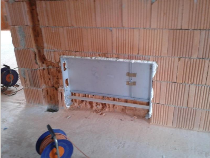
1. Installation of the distributor box
